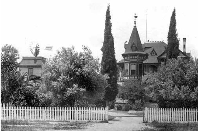
GARDEMEYER MANSION SHOWING THE TANK HOUSE.
