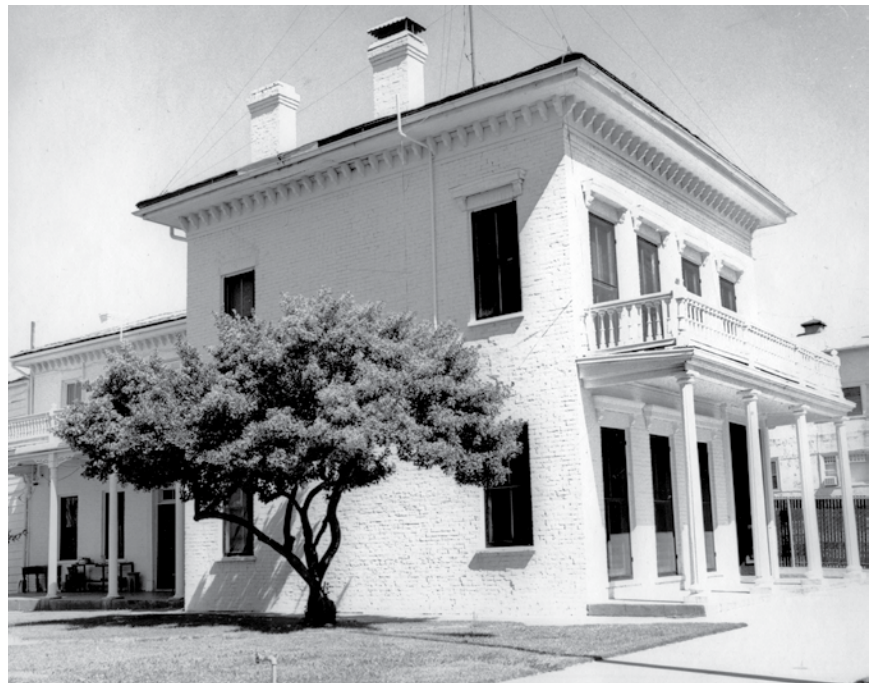
FORBES HOUSE, D STREET, MARYSVILLE.
