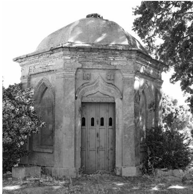
JAMES MCDONALD'S VAULT IN THE MARYSVILLE CITY CEMETERY. CONSTRUCTED IN 1871 AFTER THE DEATH OF HIS WIFE, HE JOINED HER THERE IN 1913.
