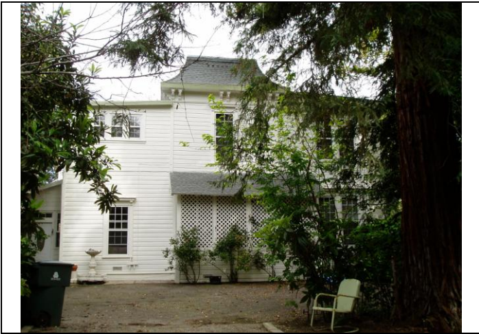
View looking east at the west elevation
