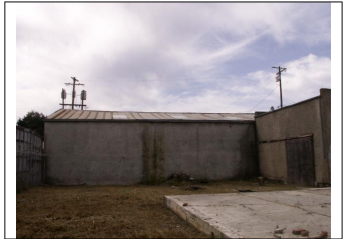
View looking south at the north elevation
