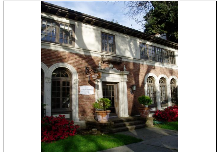
View looking northwest at the façade porch details
