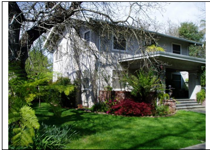
View looking west at the south elevation
