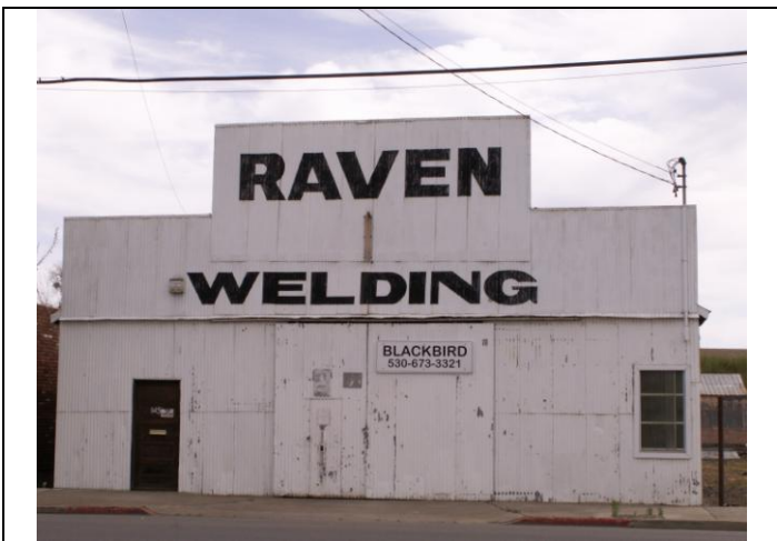
View looking east at the details on the façade
