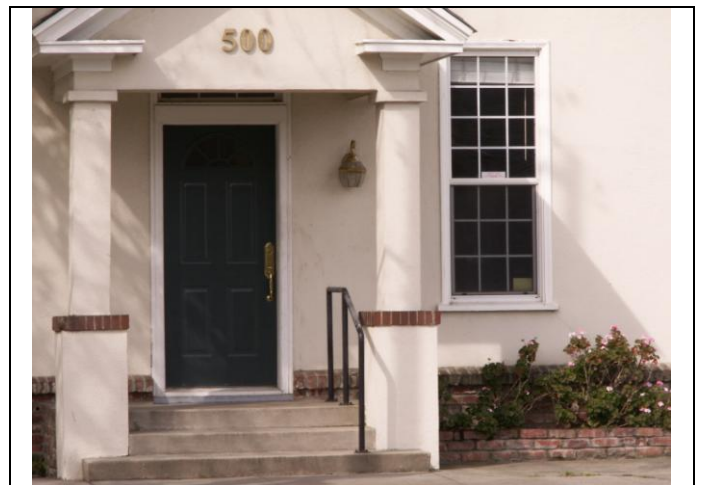
View looking west at the porch details
