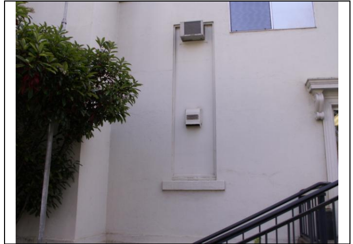
View looking east at window details on the west elevation
