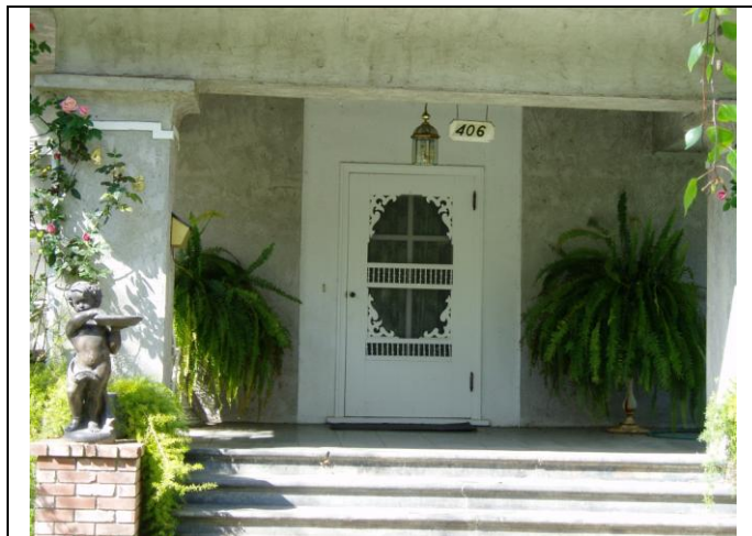
View looking at the façade porch detail
