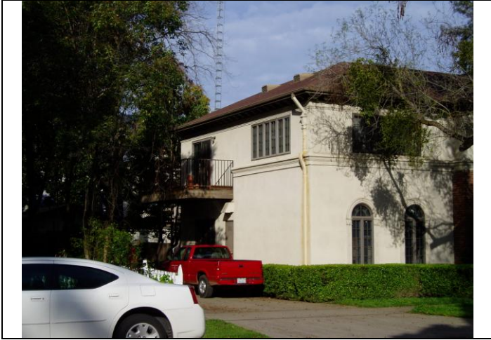
View looking northeast at the south elevation
