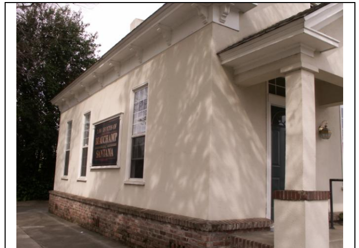
View looking northwest at the south elevation
