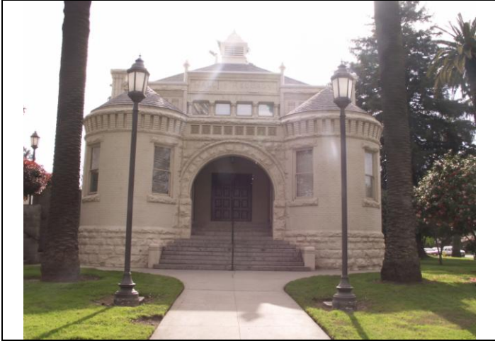
View looking west at the façade
