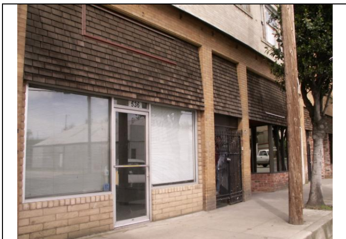
View looking northwest at the façade entry
