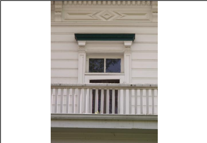
View looking east at a second floor façade detail
