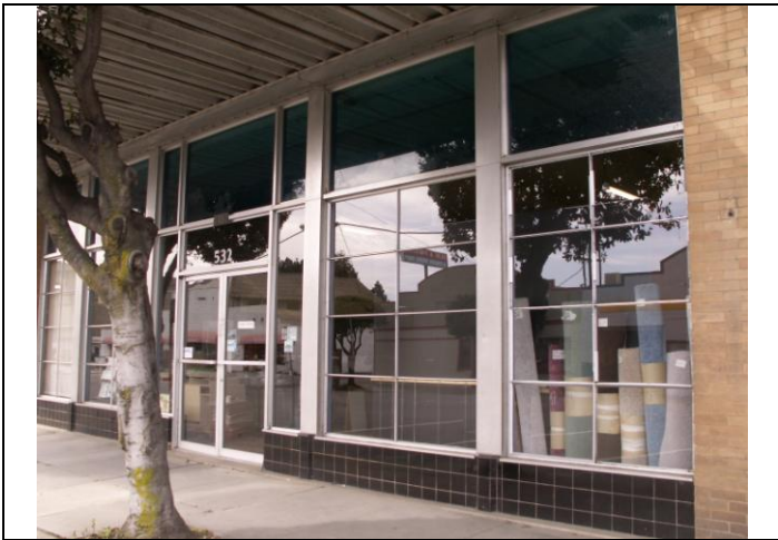
View looking south at the first floor façade
