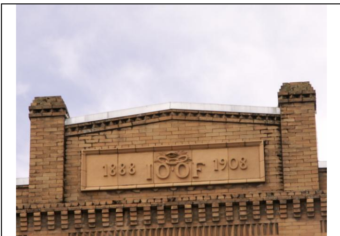
View looking west at the façade parapet
