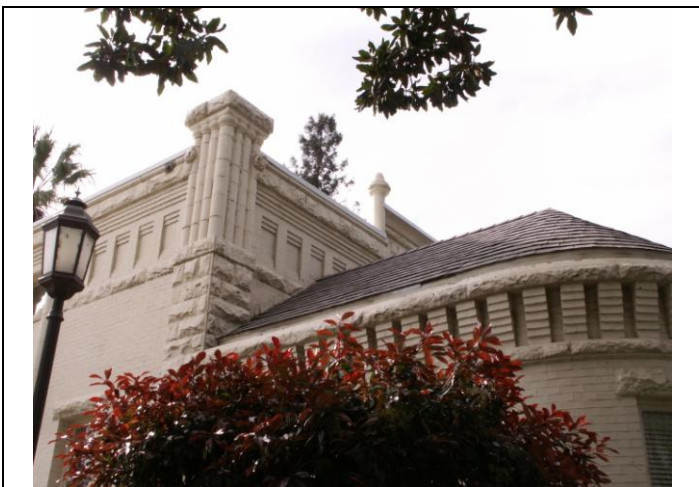
View looking northeast at the south elevation roof detail
