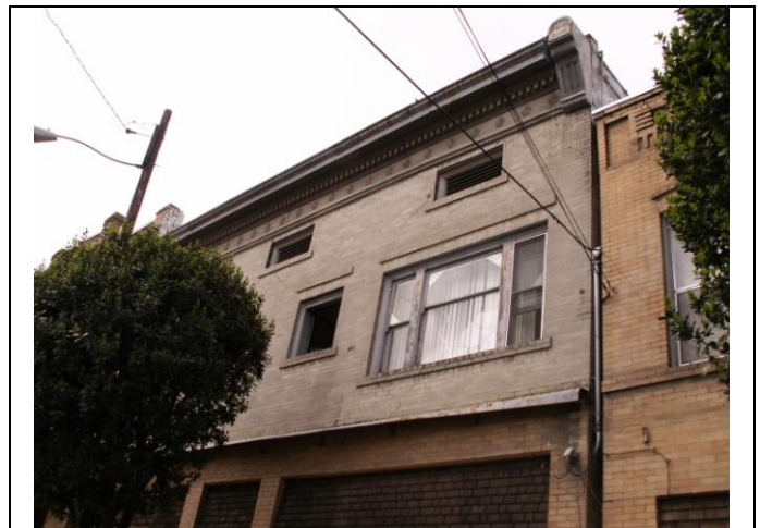
View looking southwest at the second story façade details
