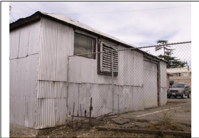
View looking southwest at the east elevation
