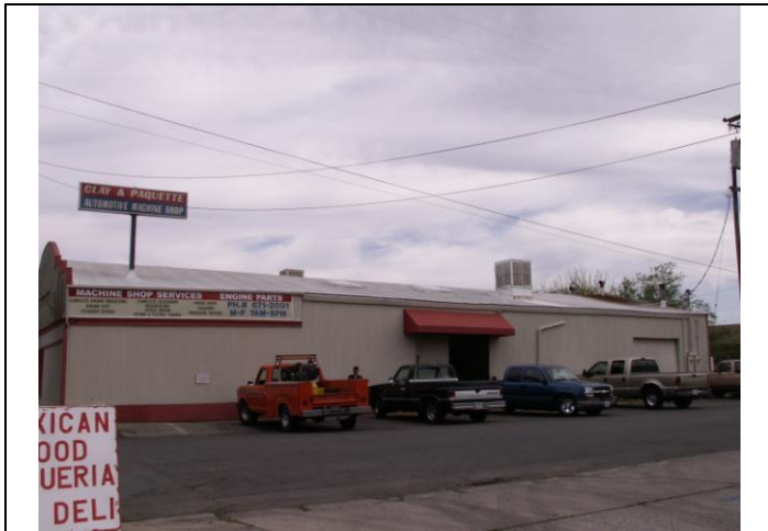
View looking northeast at the south elevation
