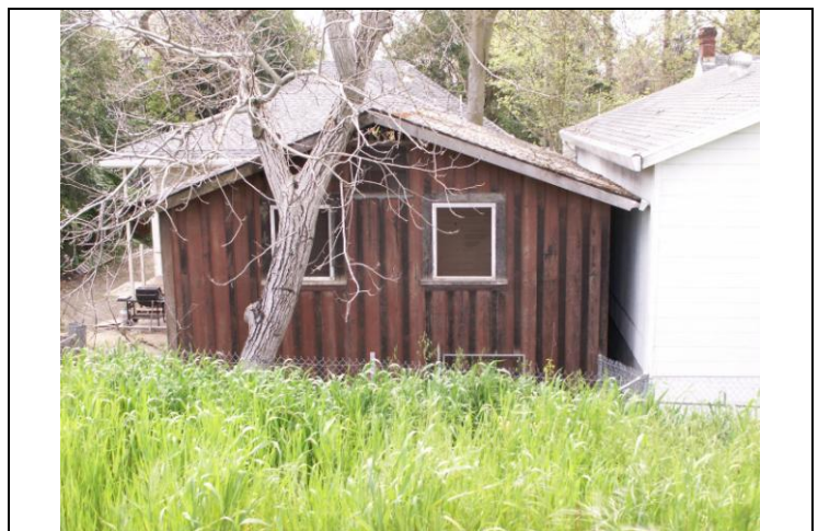
View looking west at the garage (east side) at the rear of the property
