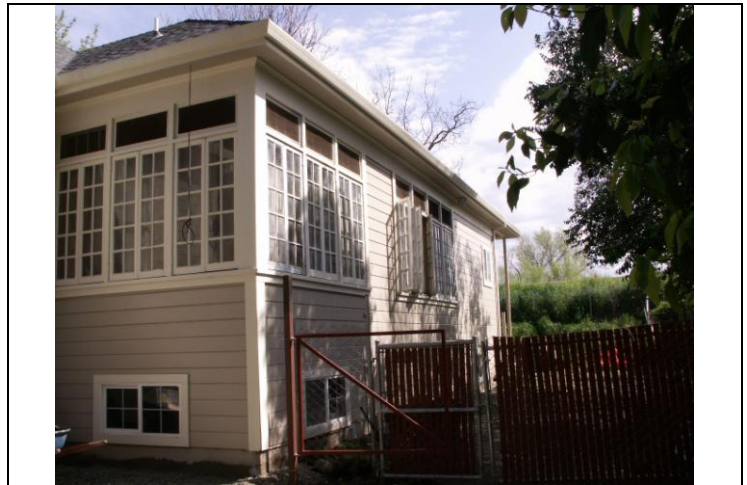
View looking northeast at the south elevation
