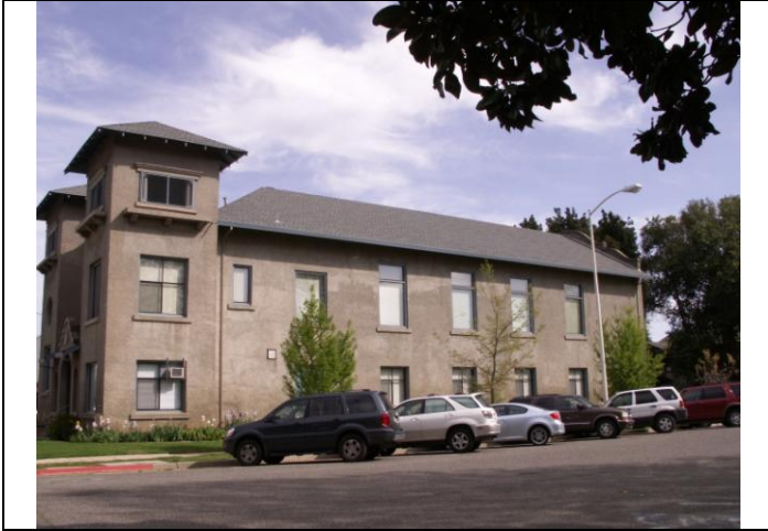
View looking northeast at the south elevation
