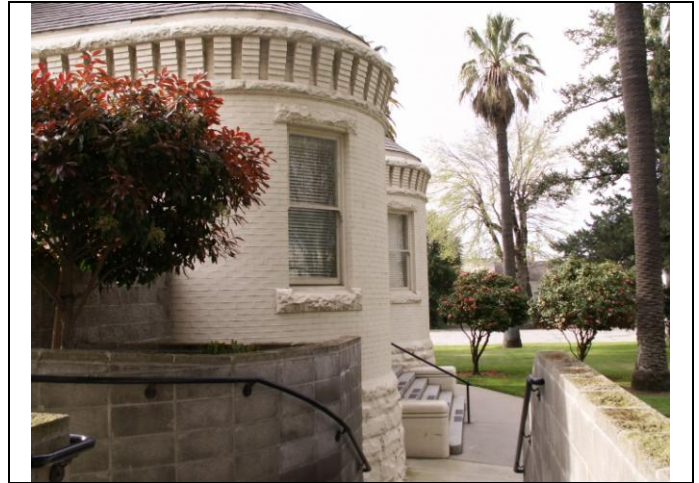
View looking north at the rounded corner of the façade and south elevation
