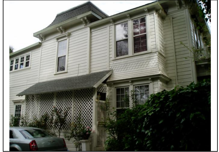
View looking north at the south elevation
