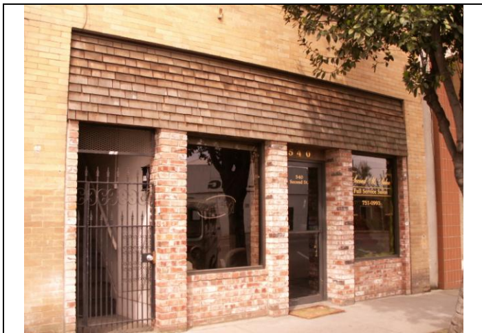
View northwest looking at the façade entry
