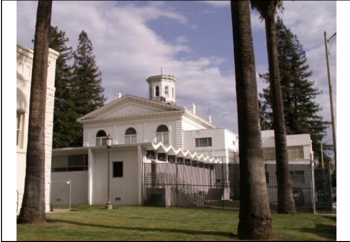
View looking south at the north elevation and addition
