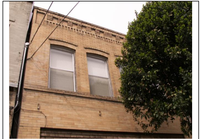
View looking northwest at the façade second story details
