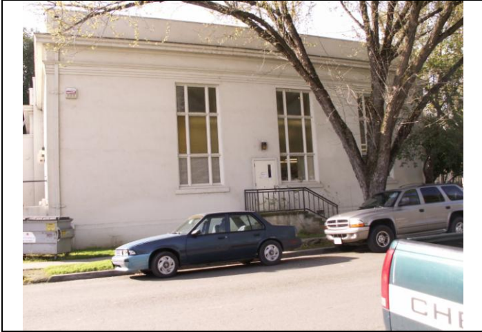
View looking south at the north elevation
