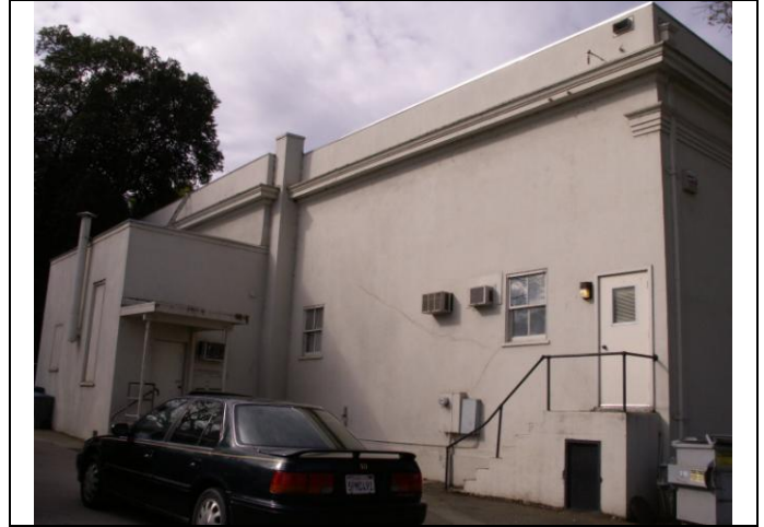
View looking southwest at the east elevation
