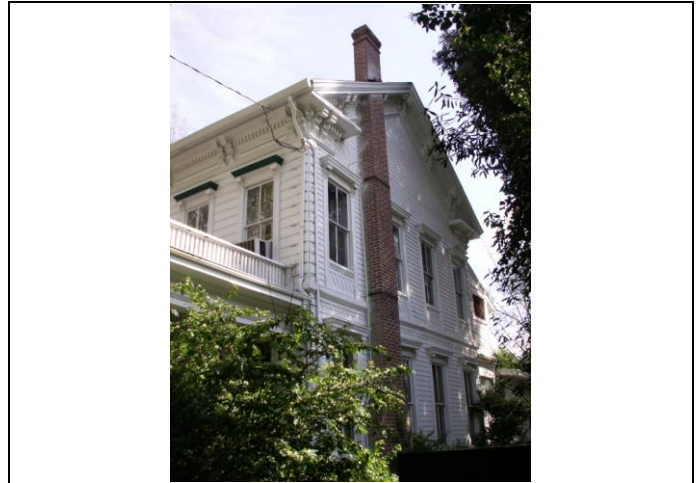
View looking northeast at the south elevation
