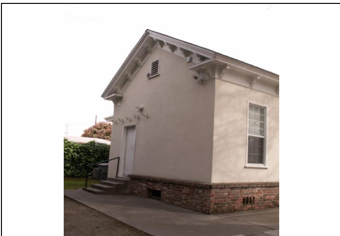
View looking northeast at the west elevation
