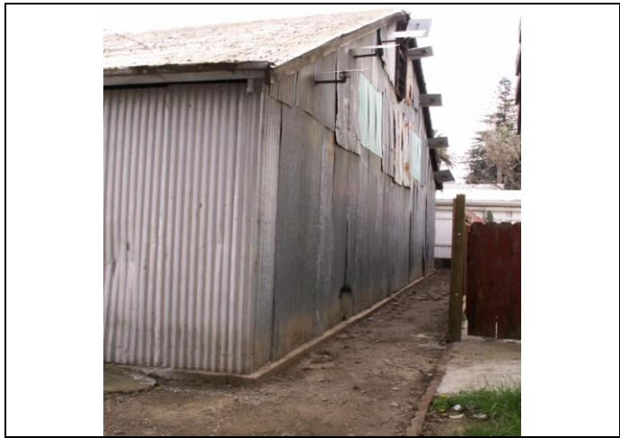
View looking south at the west elevation
