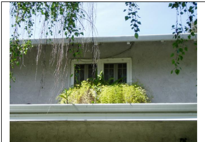
View looking at the second story window detail
