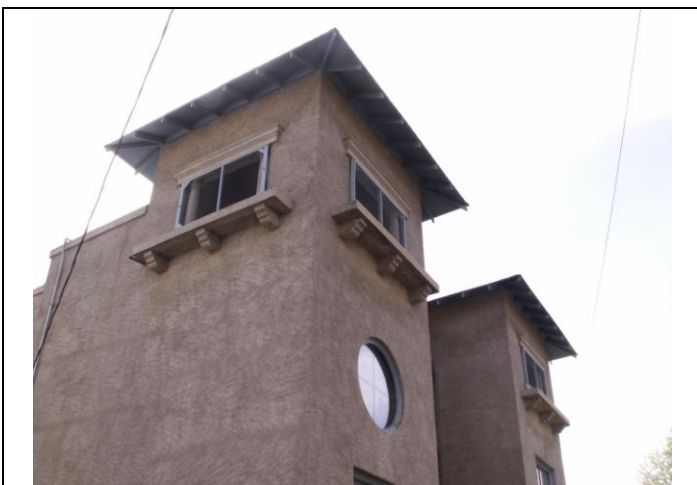
View looking southeast at the façade details
