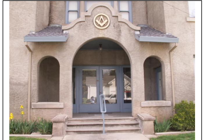
View looking east at the façade entry detail
