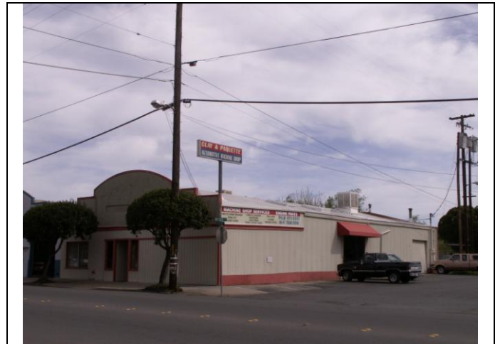
View looking northeast at the façade and south elevation
