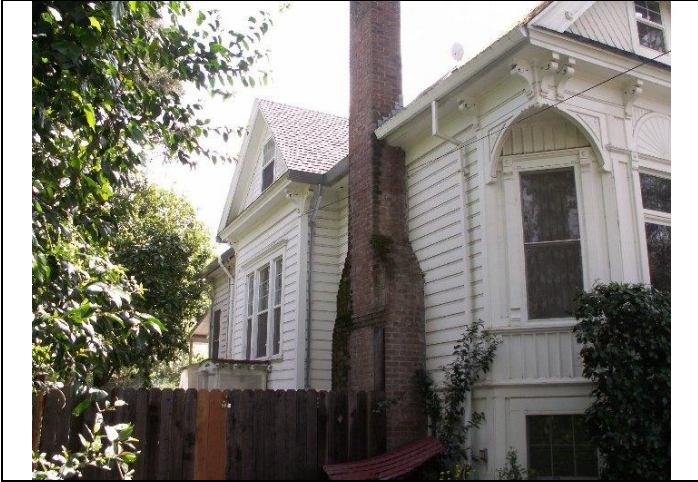
View looking southeast at the north elevation
